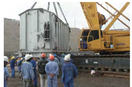
Transformer being lifted into place by Lane Cane
