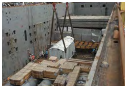
Transformers being lifted from ocean vessel cargo hold
