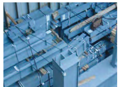
Bundles of prefabricated structural steel on the top tier adequately secured with wooden chocking and wire rope lashings
