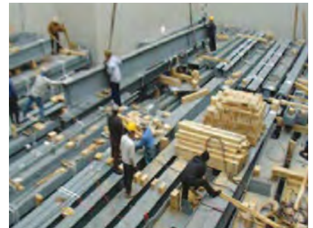
Well-stowed structural steel (fore and aft direction), with adequate dunnage between tiers
